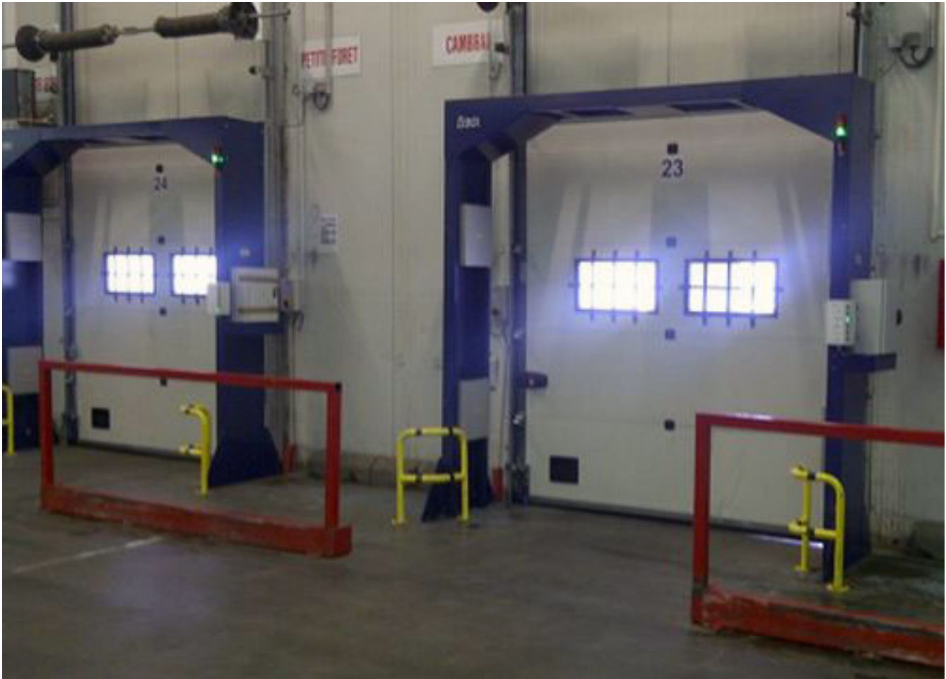
Auchan installed RFID readers alongside its loading bays' doorways, in order to record the arrival and departure of its containers.
